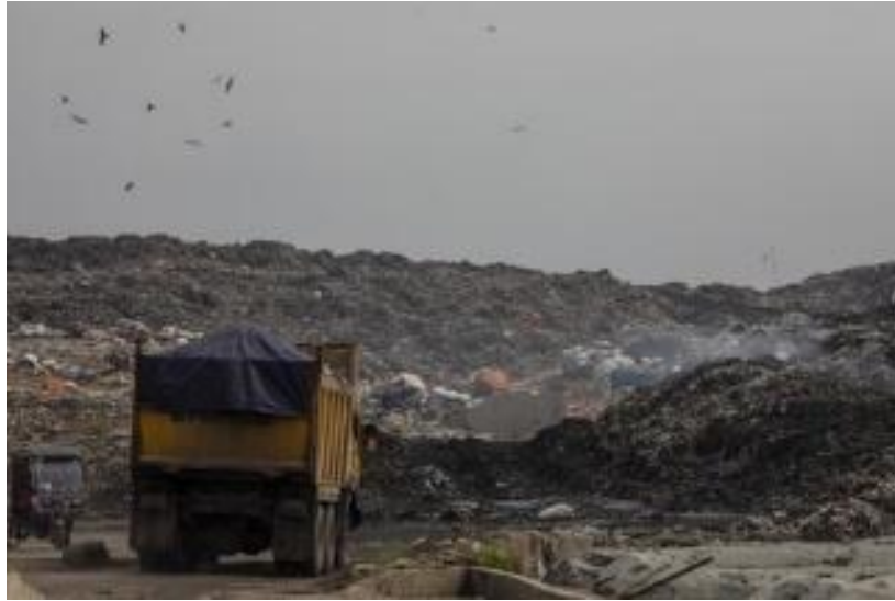
Figure 1. Waste Hill at Amin Bazar Waste Disposal Site, Source: Shutterstock
