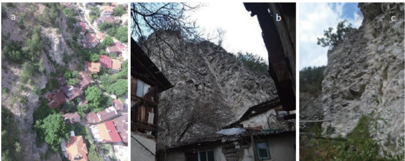
Figure 2 Images of the Rock Slope and the Houses under Threat
