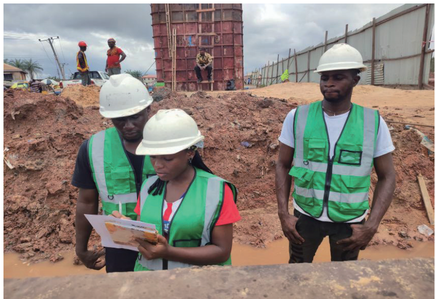
Figure 1 Author on-site for a pile load test with male colleagues
