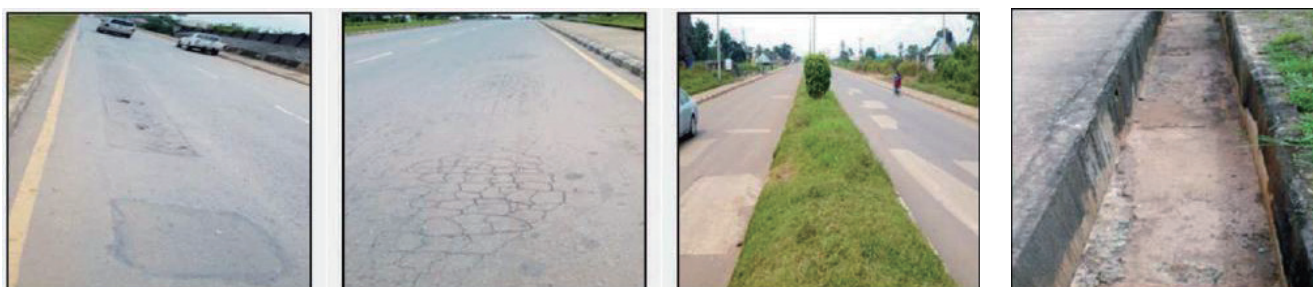
Figure 2 The Enugu – Abakaliki Road with potholes, ruts, alligator cracking, fatigue concrete & U-Shaped concrete drains (Source: Babadiya & Igwe 2021)
