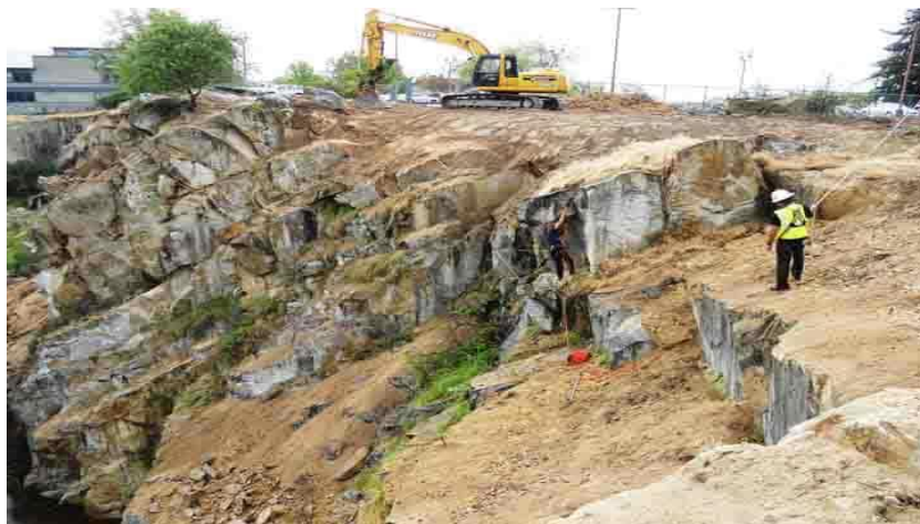
Figure 1 Engineering geologists at work on site (photo retrieved from https://www.geologypage.com/2019/04/engineering-geology.html )
