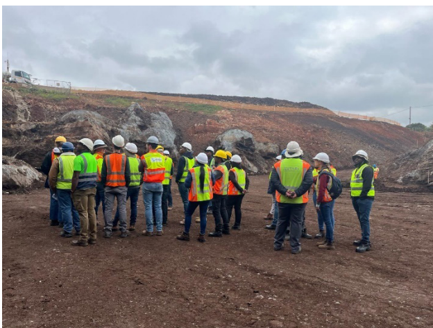
Site Visit to Sinkhole Rehabilitation on A Major Highway
