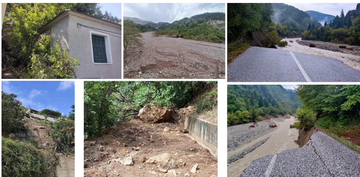
Figure 1. A number of the impacts of landslides triggered by Cyclone Daniel in the Meteora region.
