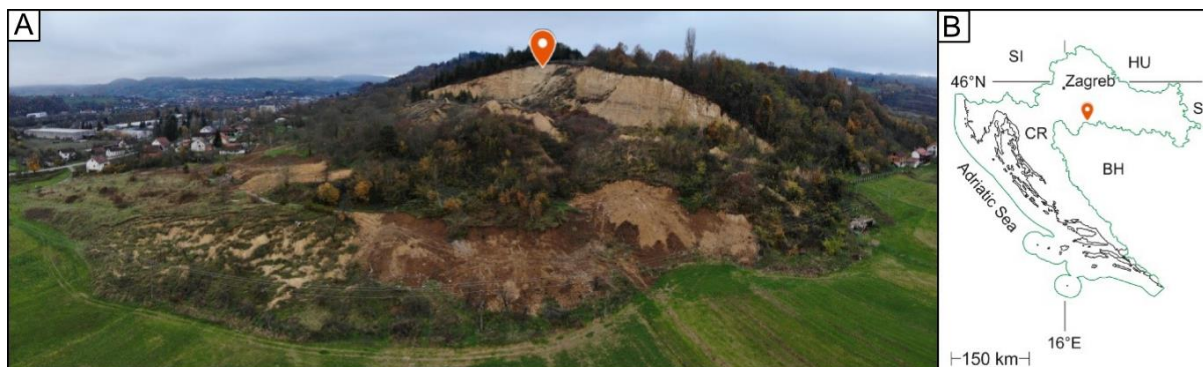
Figure 1. Hrvatska Kostajnica landslide location: A) In the city of Hrvatska Kostajnica near Una River; B) In Croatia, near the border with Bosnia and Herzegovina (red mark on the map)
