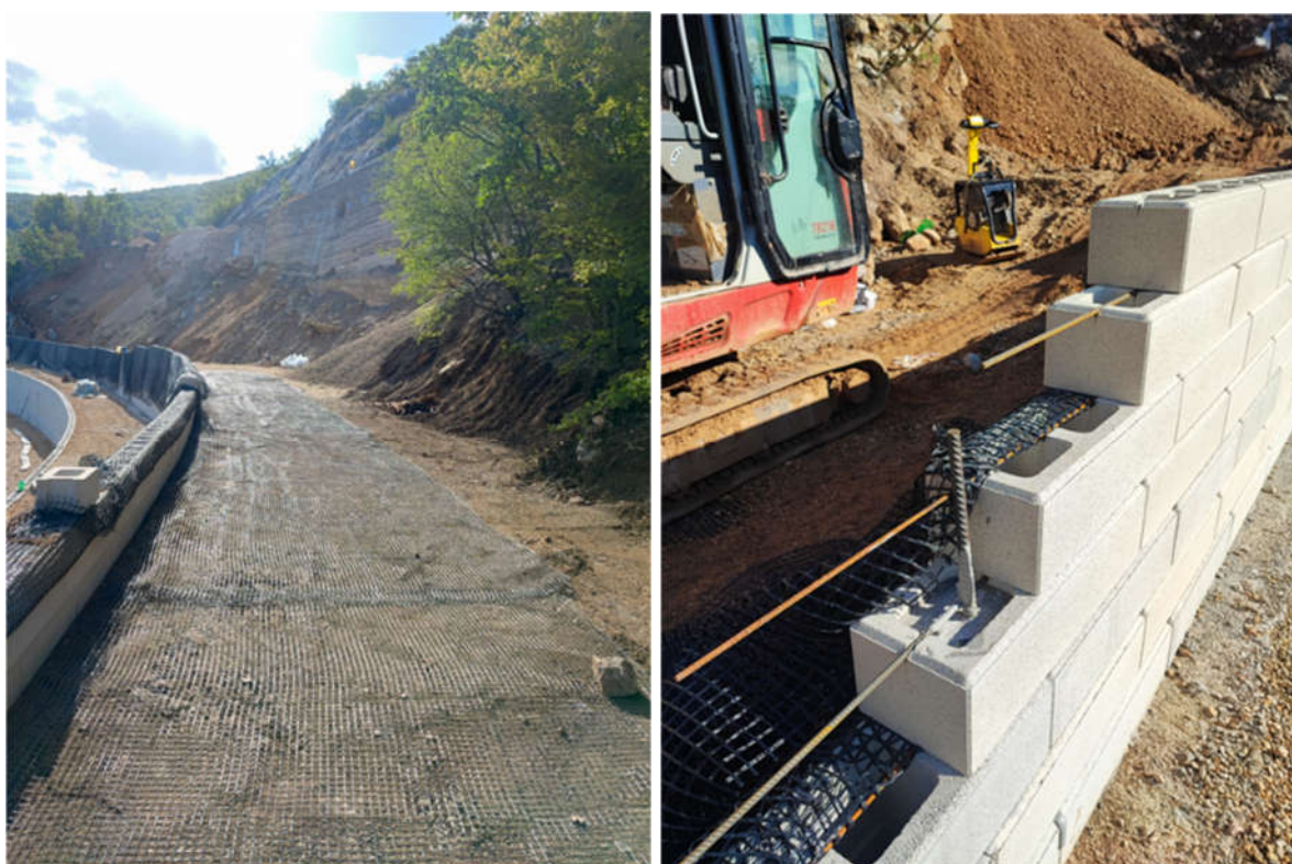
Figure 8. Reinforced earth elements
