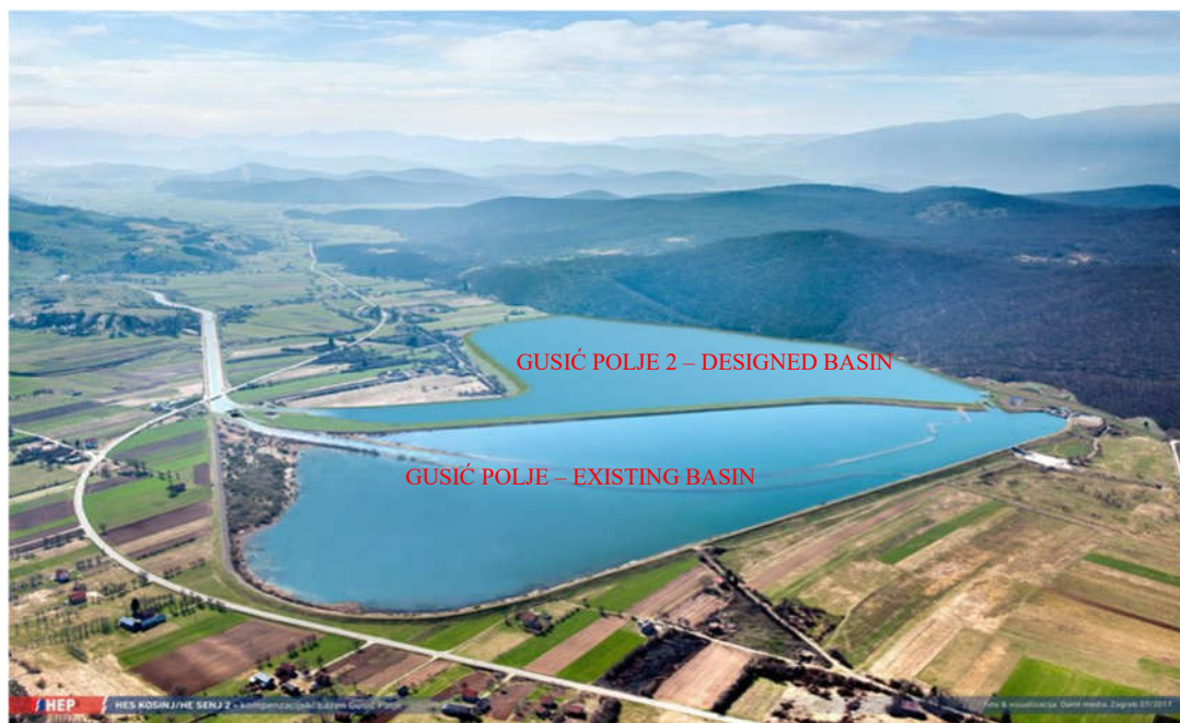
Figure 1. The broader project area showing the existing Gusić polje basin and the designed Gusić polje 2 basin
