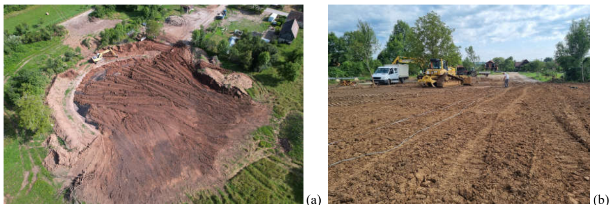
Figure 12. Installation of final layer of clay cap (a) and the terrain surface after the remediation works with SASW control quality work being conducted (right)
