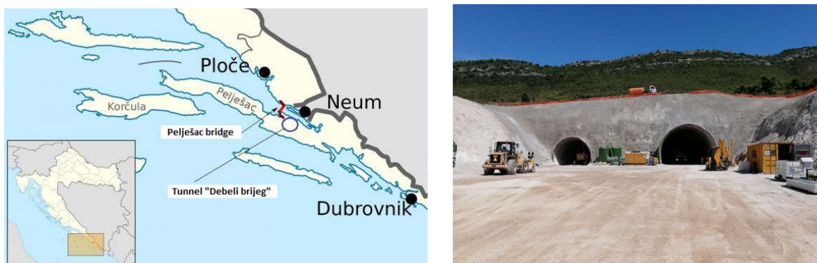
Figure 2. Tunnel "Debeli Brijeg"
