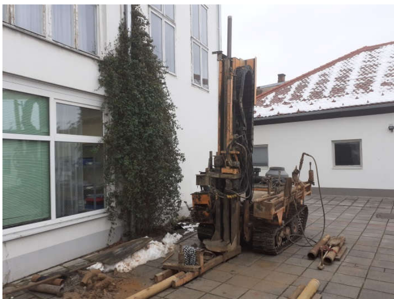
Figure 2. Location of borehole B-3 with Geotech 605D drill rig.
