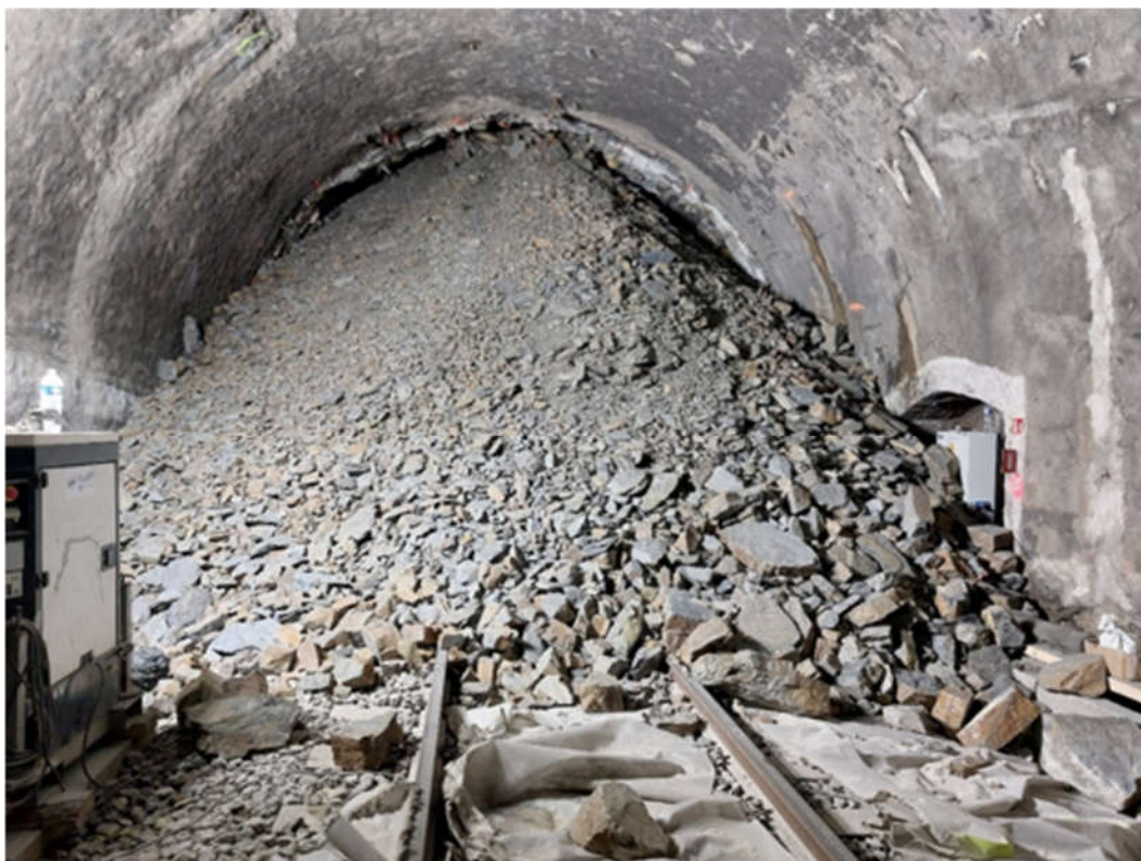
Figure 1. Rock slump seen from the southern part of the tunnel
