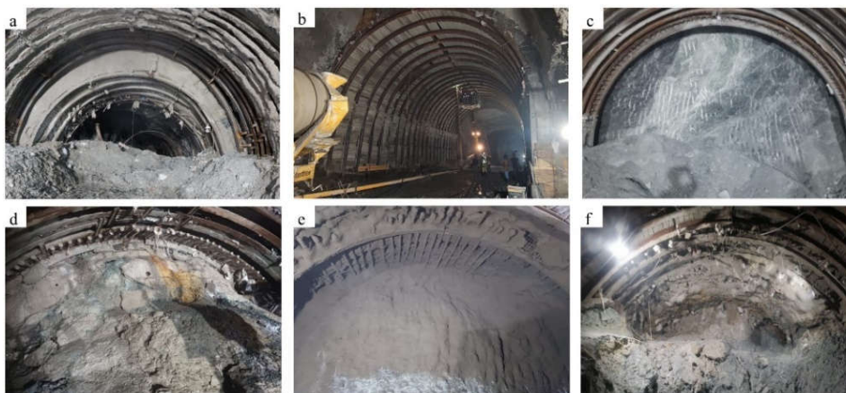
Figure 5. Showing Photographs of rectification works and additional support measures (a) restoration work under progress, skin to skin ribs were embedded under SFRS (b) Rectified tunnel (c) Fore poling to stabilise the crown of the Tunnel. (d) & (e) Pipe roofing created an umbrella-like structure above the crown to prevent collapses. (f) Multisegmental excavation.
