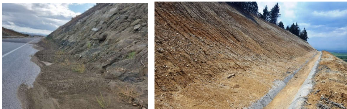
Figure 1. Slope exposed to intensive erosion on the Highway Miladinovci – Shtip, N. Macedonia.
