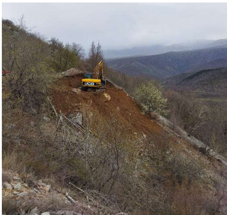
Figure 5. The beginning of the construction of the access road
