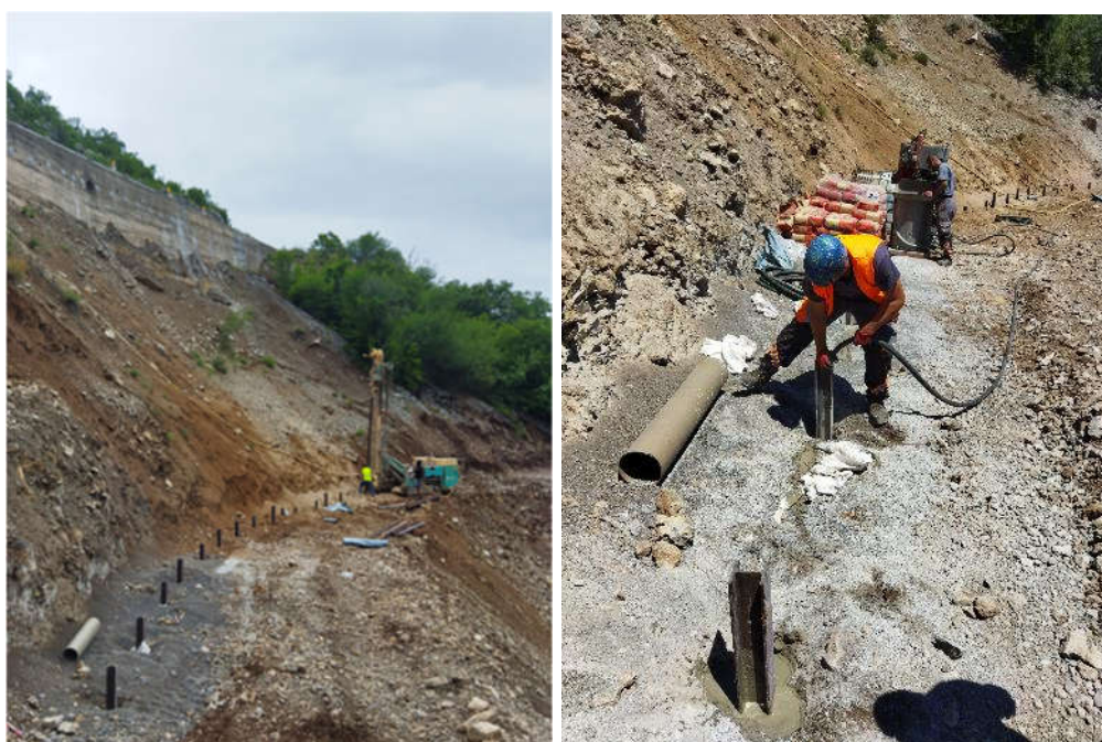
Figure 6. Installation of micropiles
