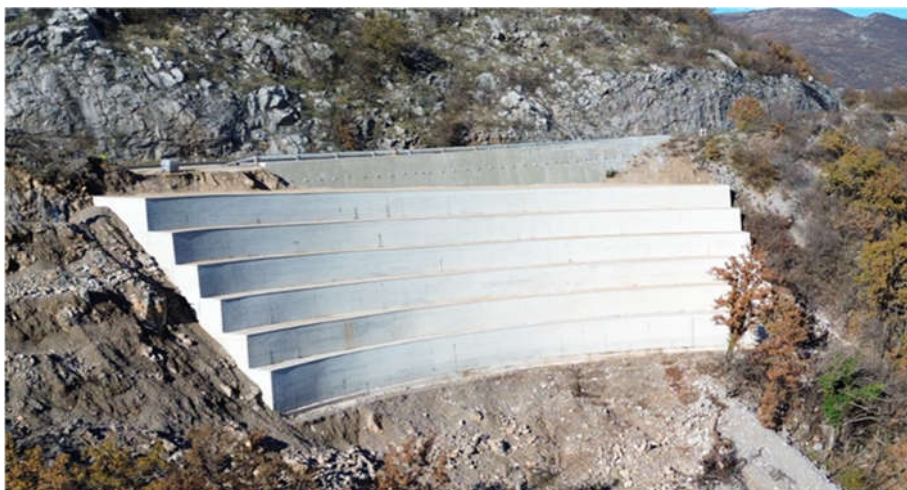
Figure 9. Completed construction, October 2023
