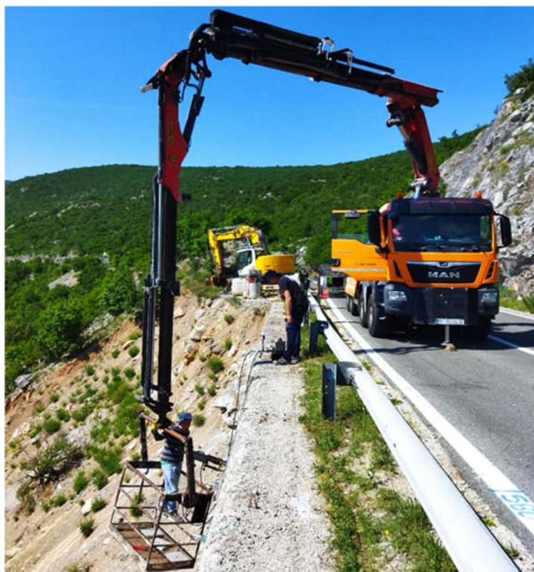
Figure 4. Installing of rock anchors
