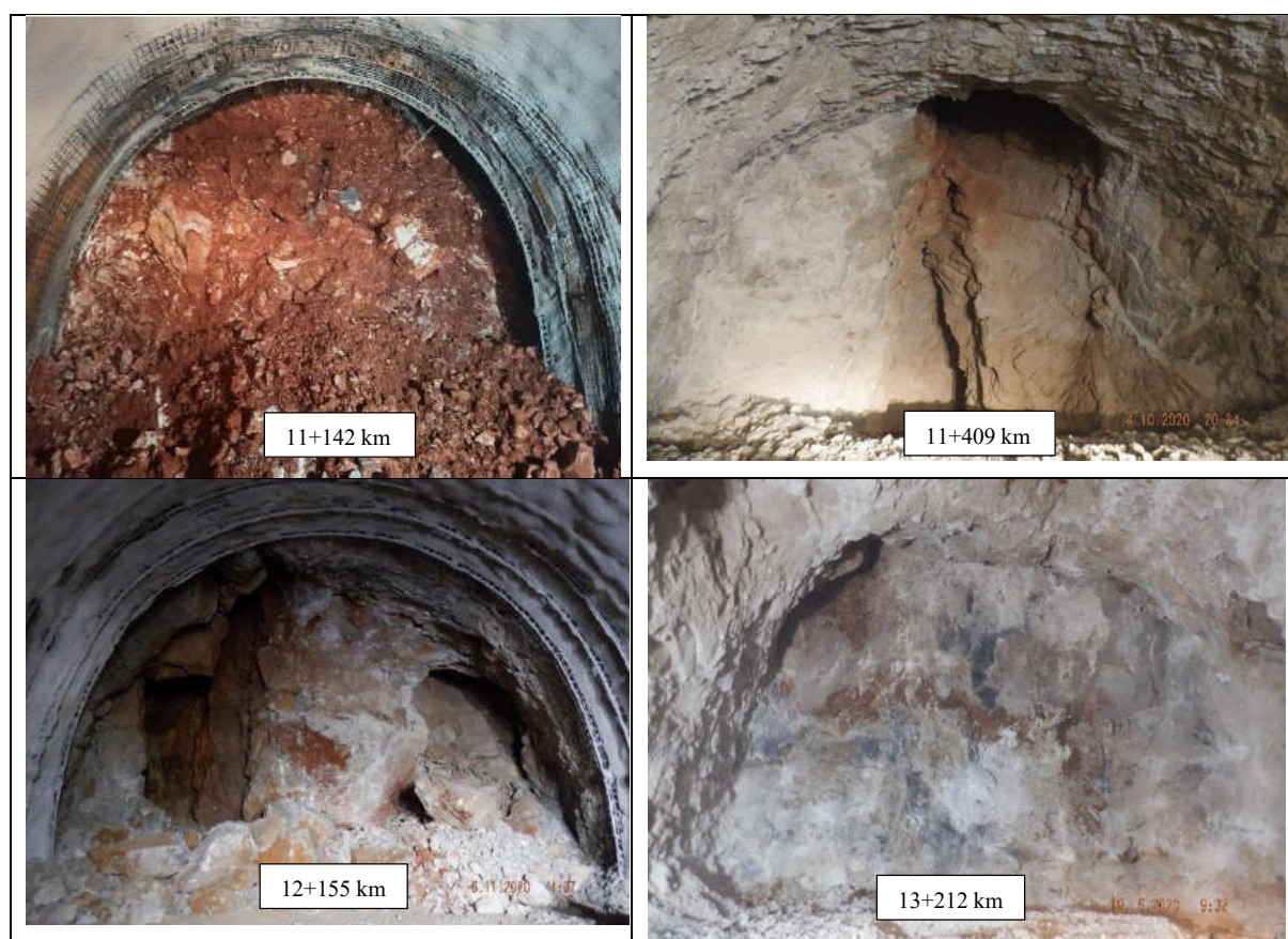
Figure 7. Tunnel Debeli brijeg (Pelješac peninsula)
