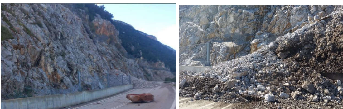
Figure 3. Falling of an individual boulder of 8m 3 (maximum boulder size of the rockfall) that bounced off the existing protection measures and ended up on the road deck within the provincial road, at about Ch. 5+525 km. Close-up view of debris flow (on the right)
