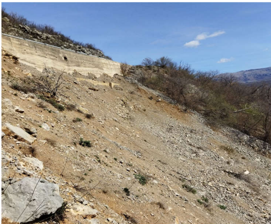
Figure 1. The initial state of the landslide, March 2023
