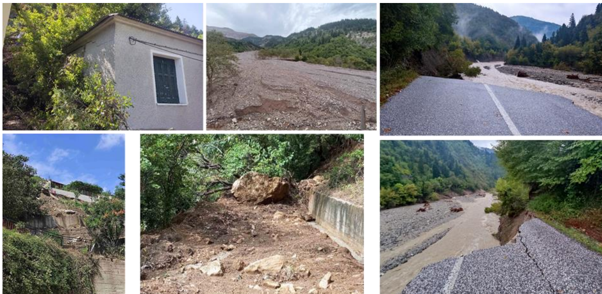
Figure 1. A number of the impacts of landslides triggered by Cyclone Daniel in the Meteora region.
