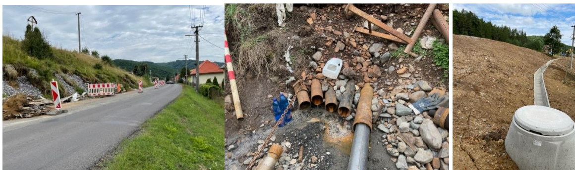
Figure 1. From left – outlet of prefabricated drains at the foot of the landslide; realization of horizontal drainage wells; surface rigol and control shaft
