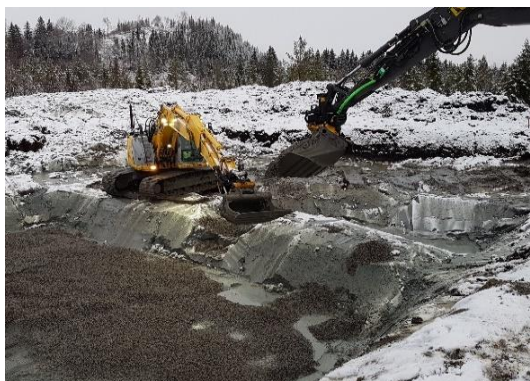
Figure 1. Two excavators spreading crushed stone into the excavation pit
