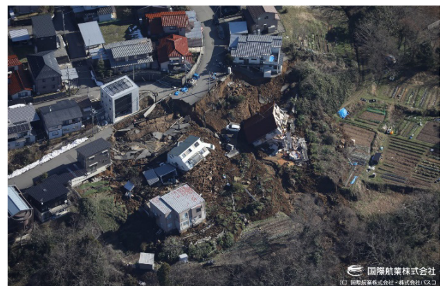
Fig. 5. Damage to buildings in Tagamishinmachi, Kanazawa City, Ishikawa Prefecture
