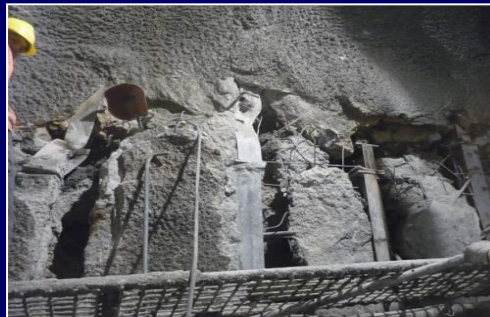
Damage of linings
