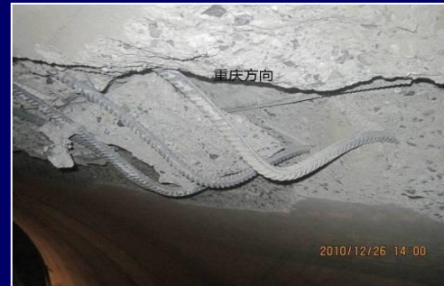
Damage of linings
