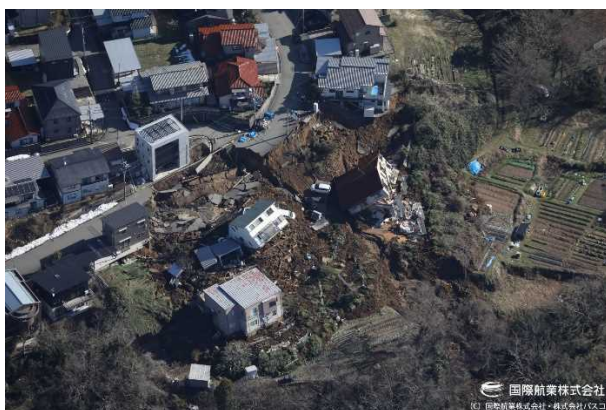
Fig. 9. Damage to buildings in Tagamishin-machi, Kanazawa City, Ishikawa Prefecture
