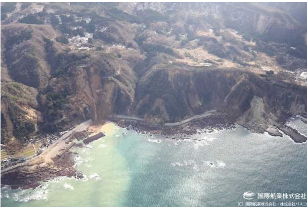
Fig. 11. Collapse of slope along Route 249, Matsunagi-machi, Suzu City, Ishikawa Prefecture
