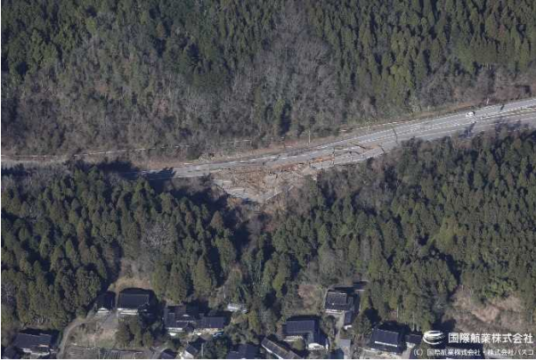
Fig. 10. Damage to the Noto Satoyama Kaido Road, that directly connects Kanazawa City to the Noto Peninsula, Ishikawa Prefecture
