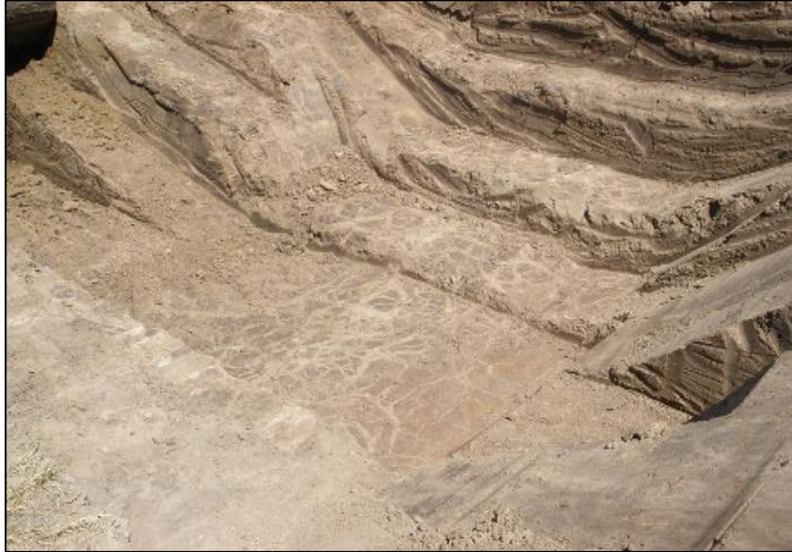
Figure 9. Cracked reactive soils between pipeline inverts
