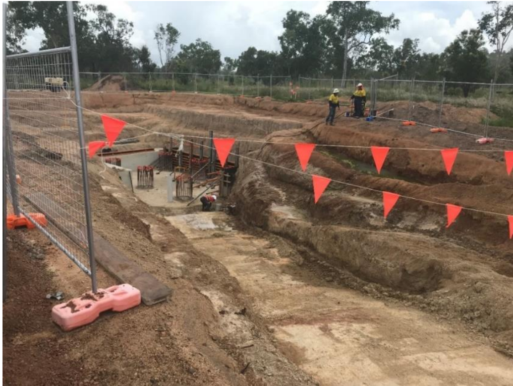
Figure 13. Large excavation & piling required for a railway underbore of a large diameter GFRP water pipeline
