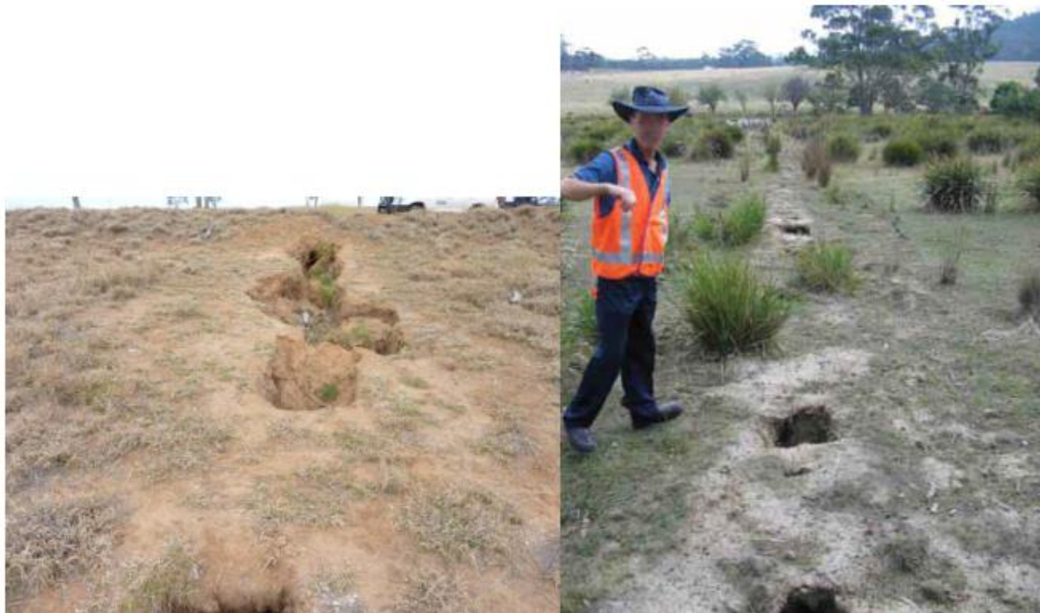
Figure 11. Typical Tunnel Erosion of Over Pipeline Backfilled Alignments
