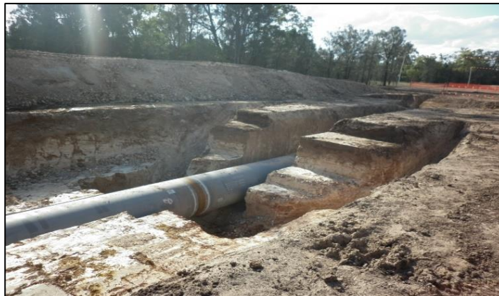
Figure 6. Gas pipeline installed in a silcrete subsurface profile, West Queensland
