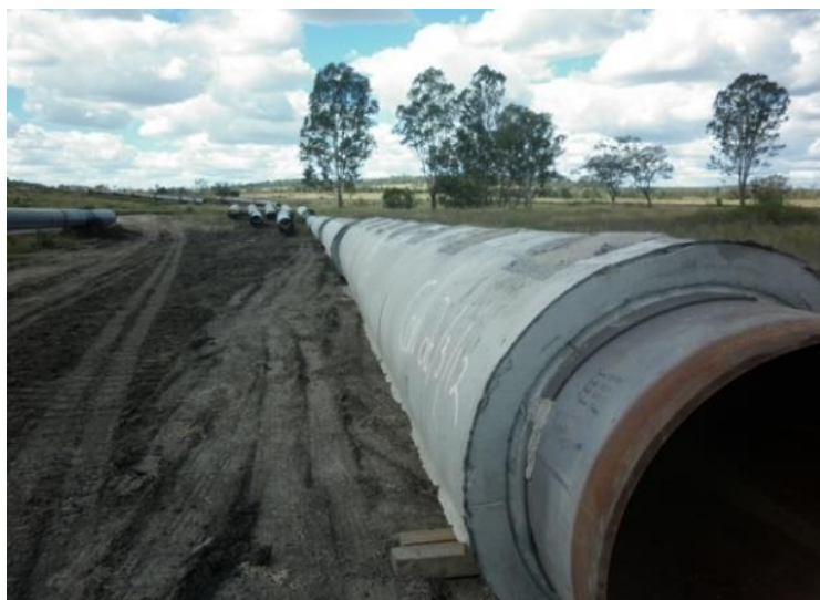
Figure 7. Concrete Lining on Steel Pipe
