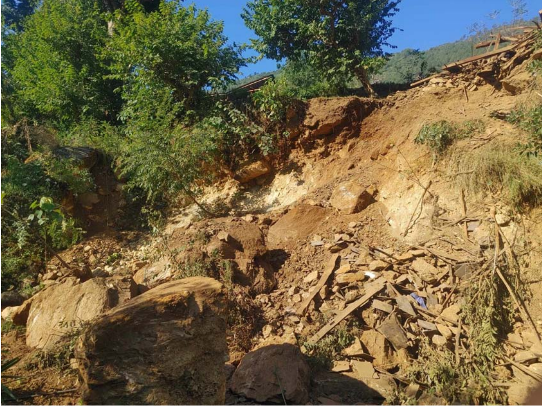
Figure 8, Landslide triggered by Jajarkot Earthquake, Nalgad Municipality
