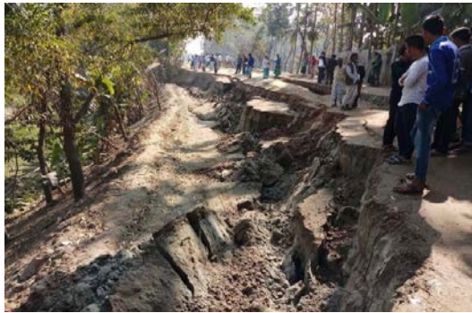
Figure 1: Road collapse between Kapasia-Sreepur on 13 February 2018 Photo credit: The Daily Asian Age
