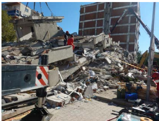
Totally collapsed and damaged eight storey buildings
