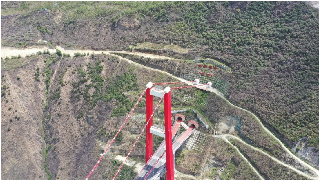
Fig. 5 After the completion of construction on the left bank
