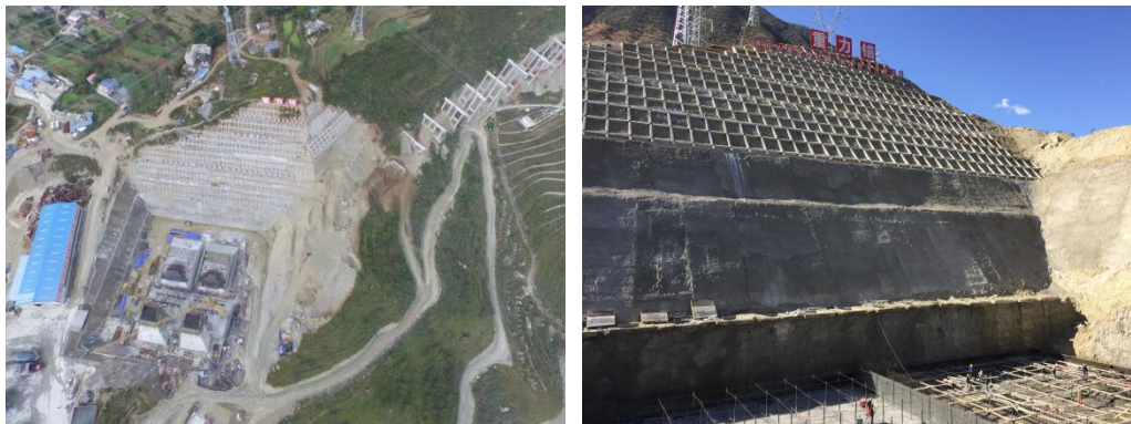
Fig. 8 Construction of the Deep Foundation Pit for the Gravity Anchor
