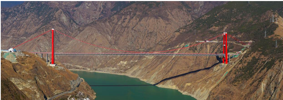
Fig. 1 Overview of Yakang Bridge
