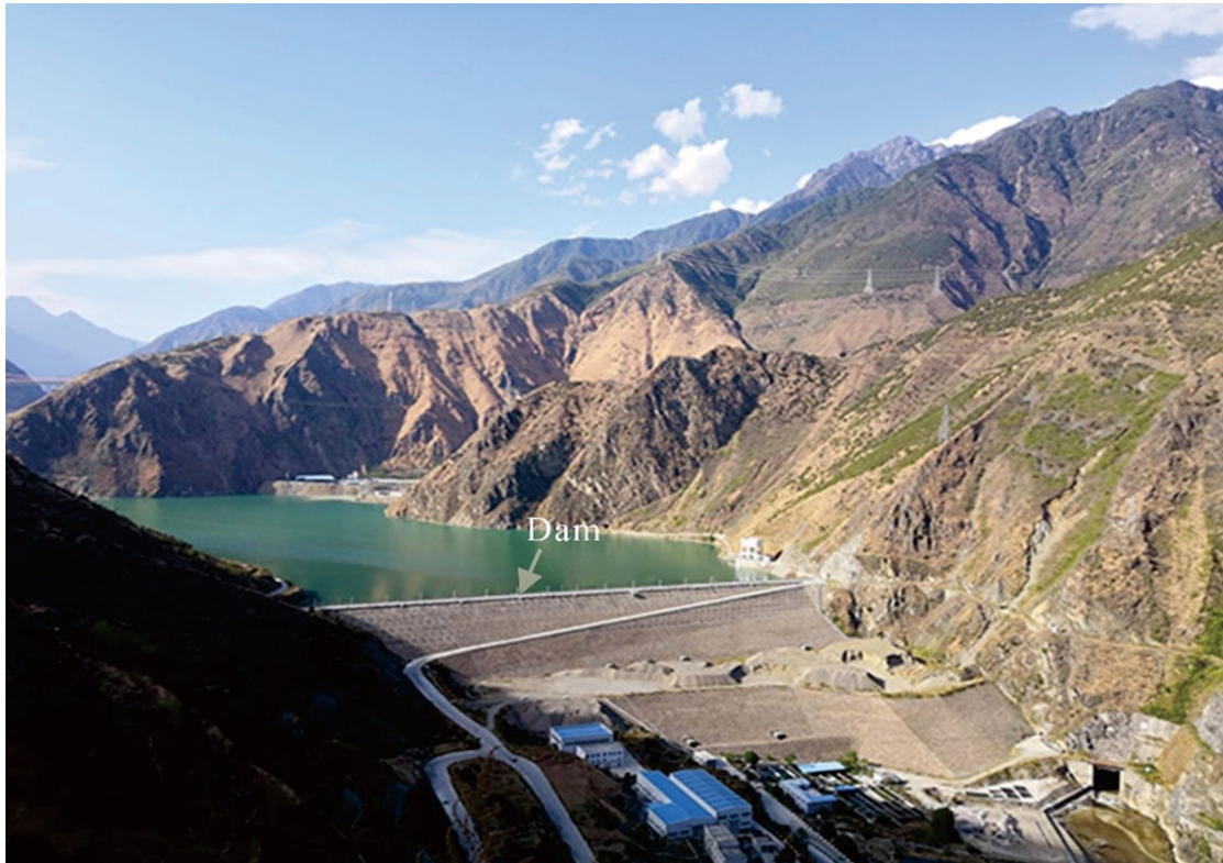
Fig. 1 Luding Hydropower Station
