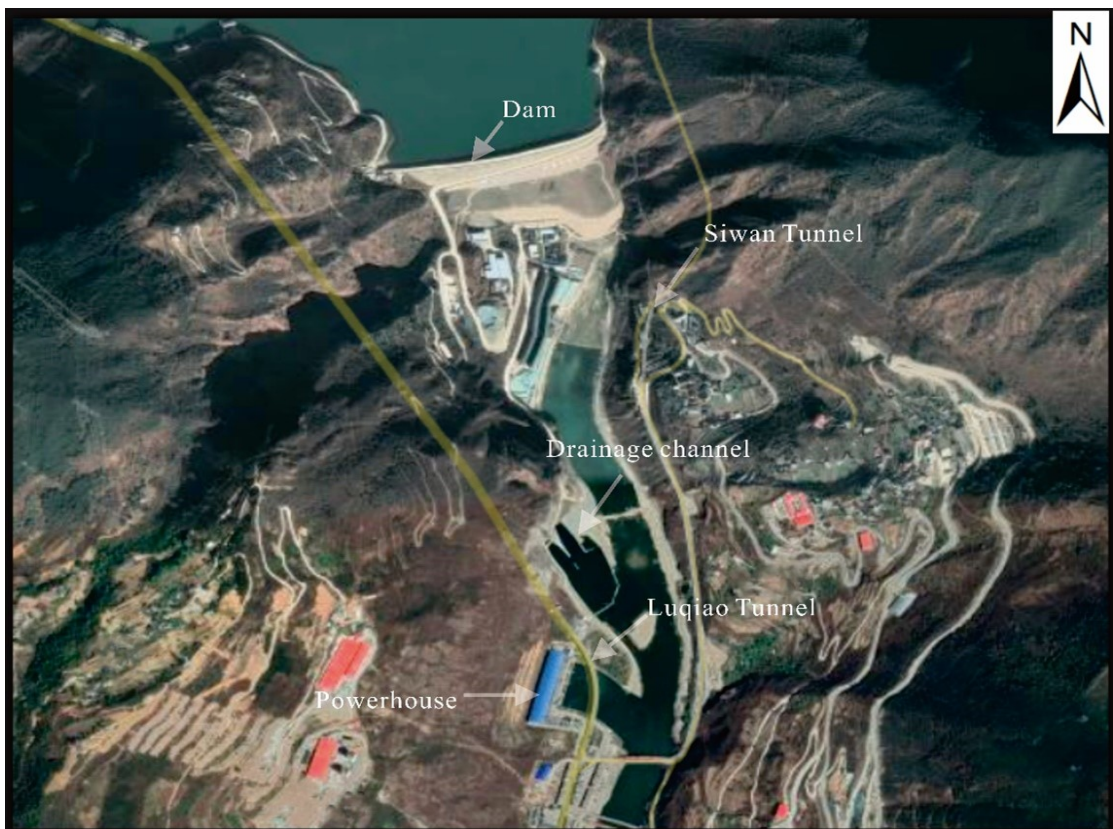
Fig. 2 Luding Hydropower Station
