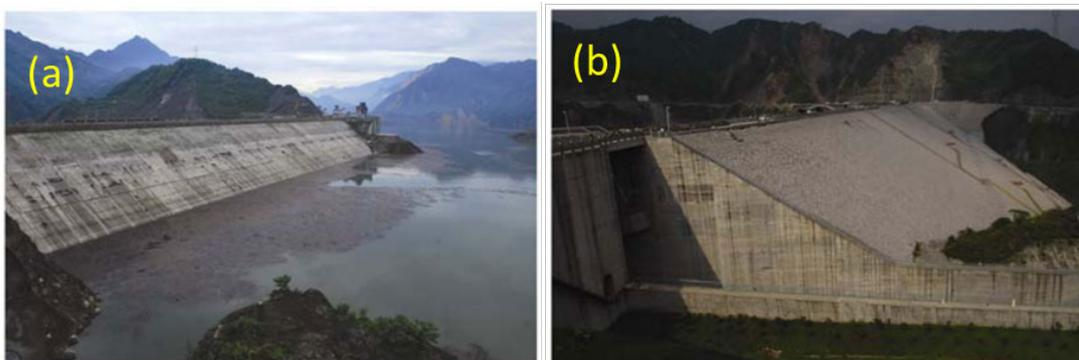
**Fig.10 Zipingpu Dam after the May 12 earthquake. (a) Upstream slabs (reservoir level 830.0 m). (b) Downstream slope of the dam and the open channel spillway.**
