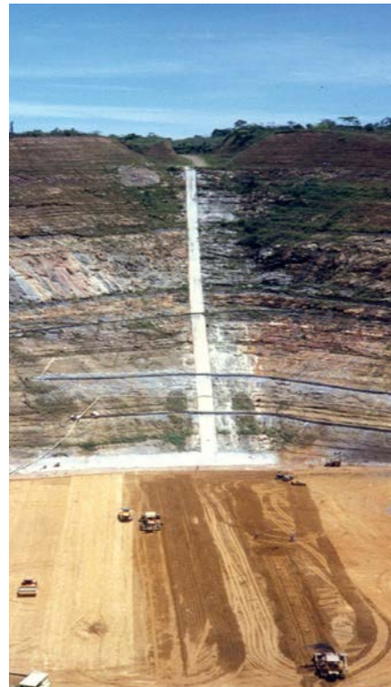
Borde Seco dam (Venezuela), under construction late eighties
