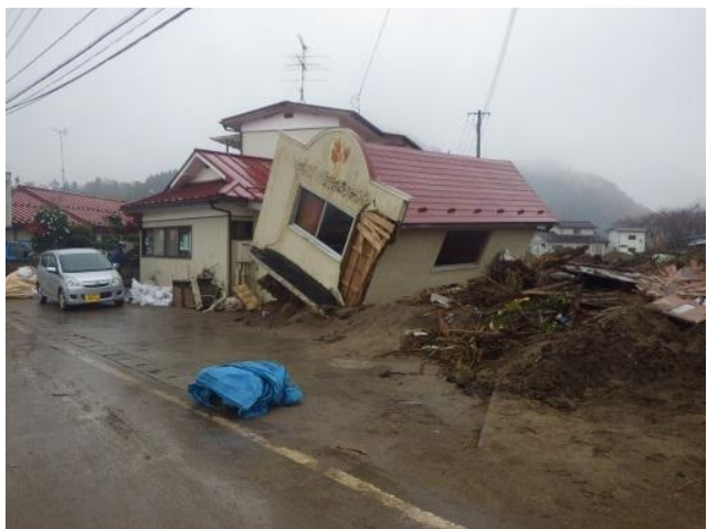
Damaged building by debris flow at Marumori-machi, Miyagi pref.
