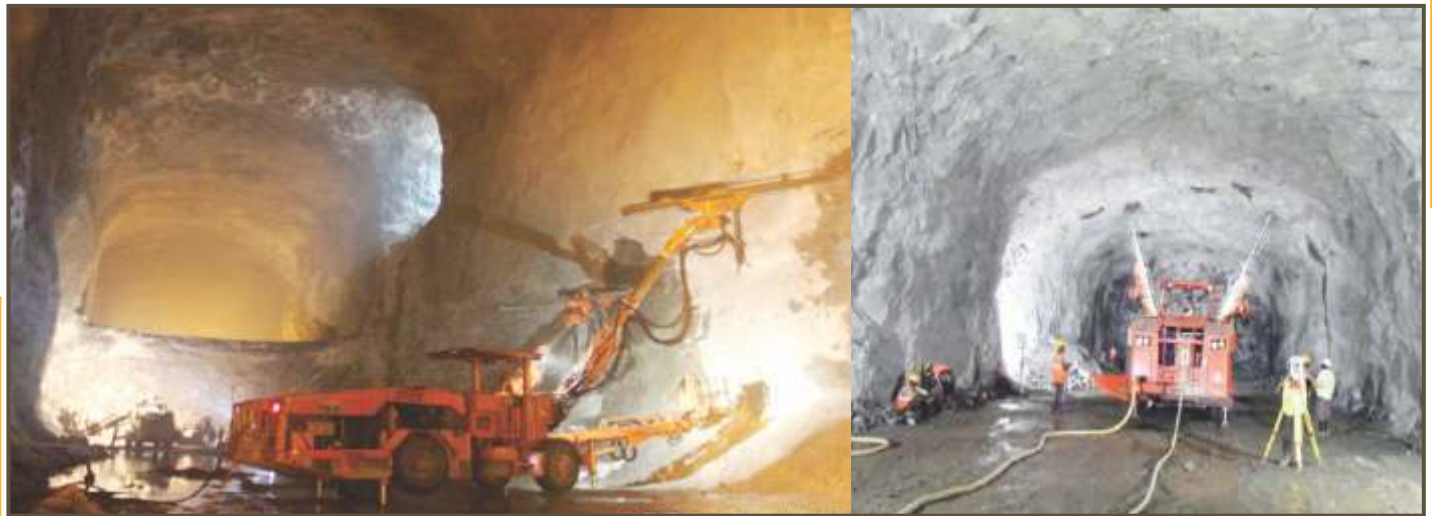
Figure 9.11: Typical rock bolt installation on wall & roof of caverns
