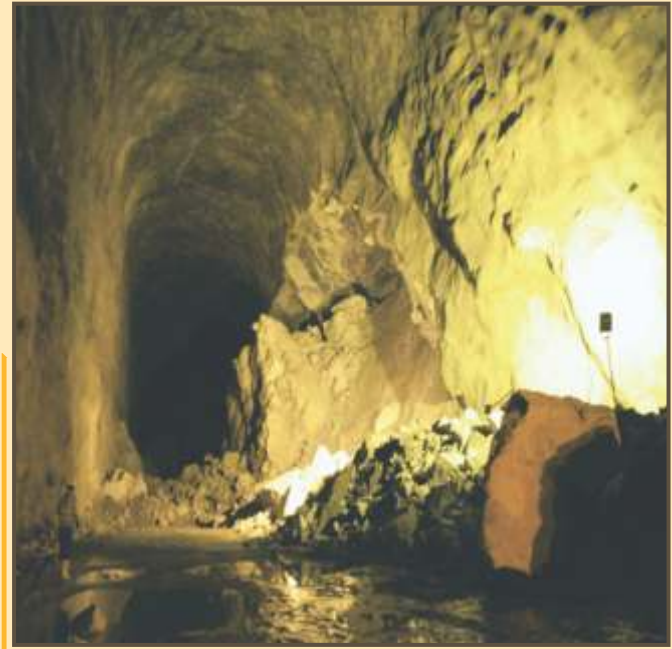
Figure 6.5: Pictorial view of the cavern failure
