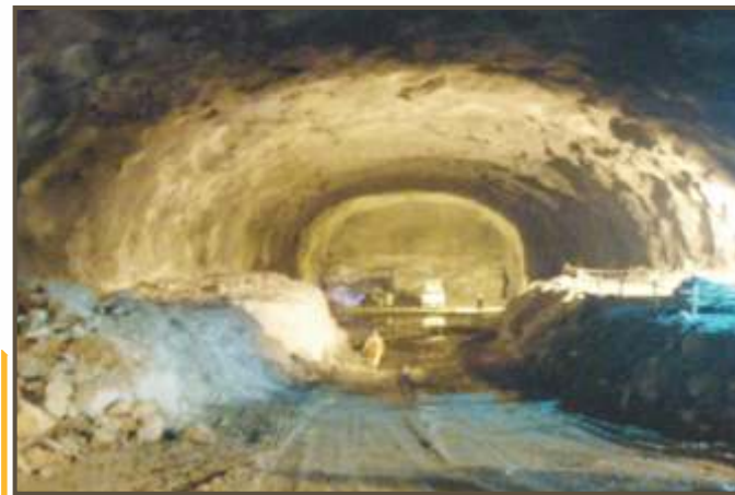
Figure 9.6: Cavern heading & bench excavation
