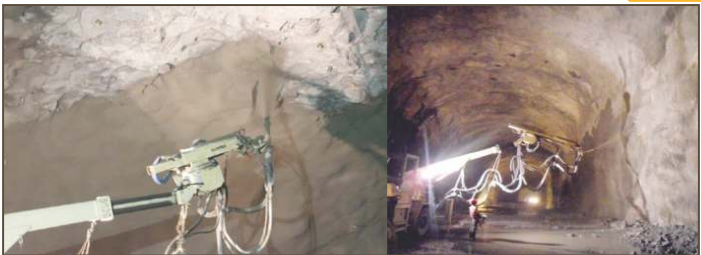
Figure 9.12: Shotcreting of cavern wall & roof in progress
