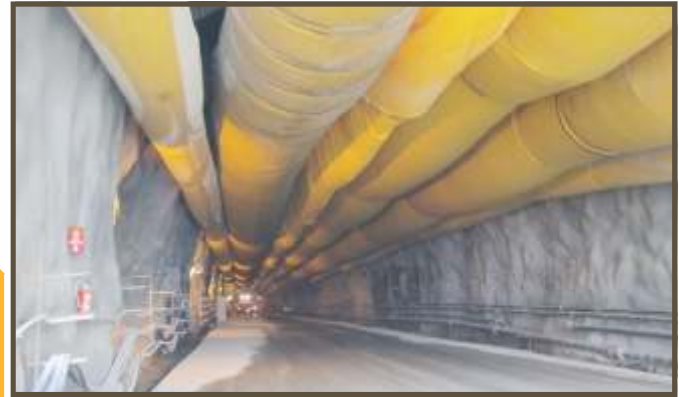
Figure 9.14: Ventilation ducts inside access tunnel
