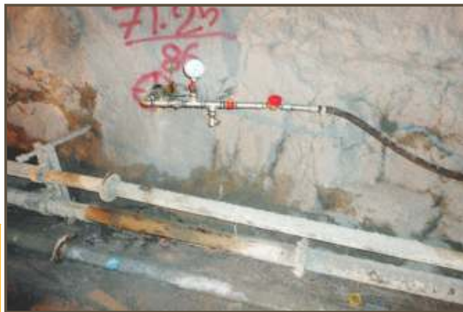
Figure 9.5: Temporary pressurization system for WC boreholes
