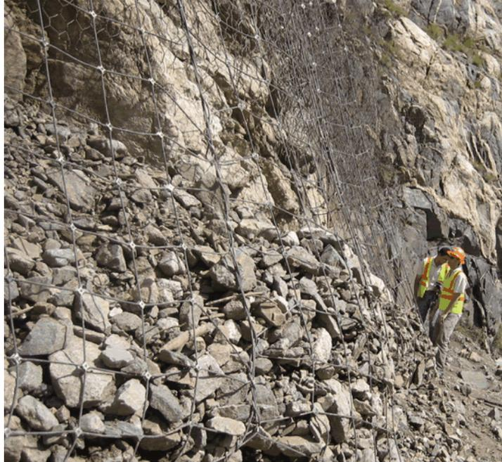
**Figure 21. Photo. Rockfall Fence Containing an Overflow of Rock Fragments.**
