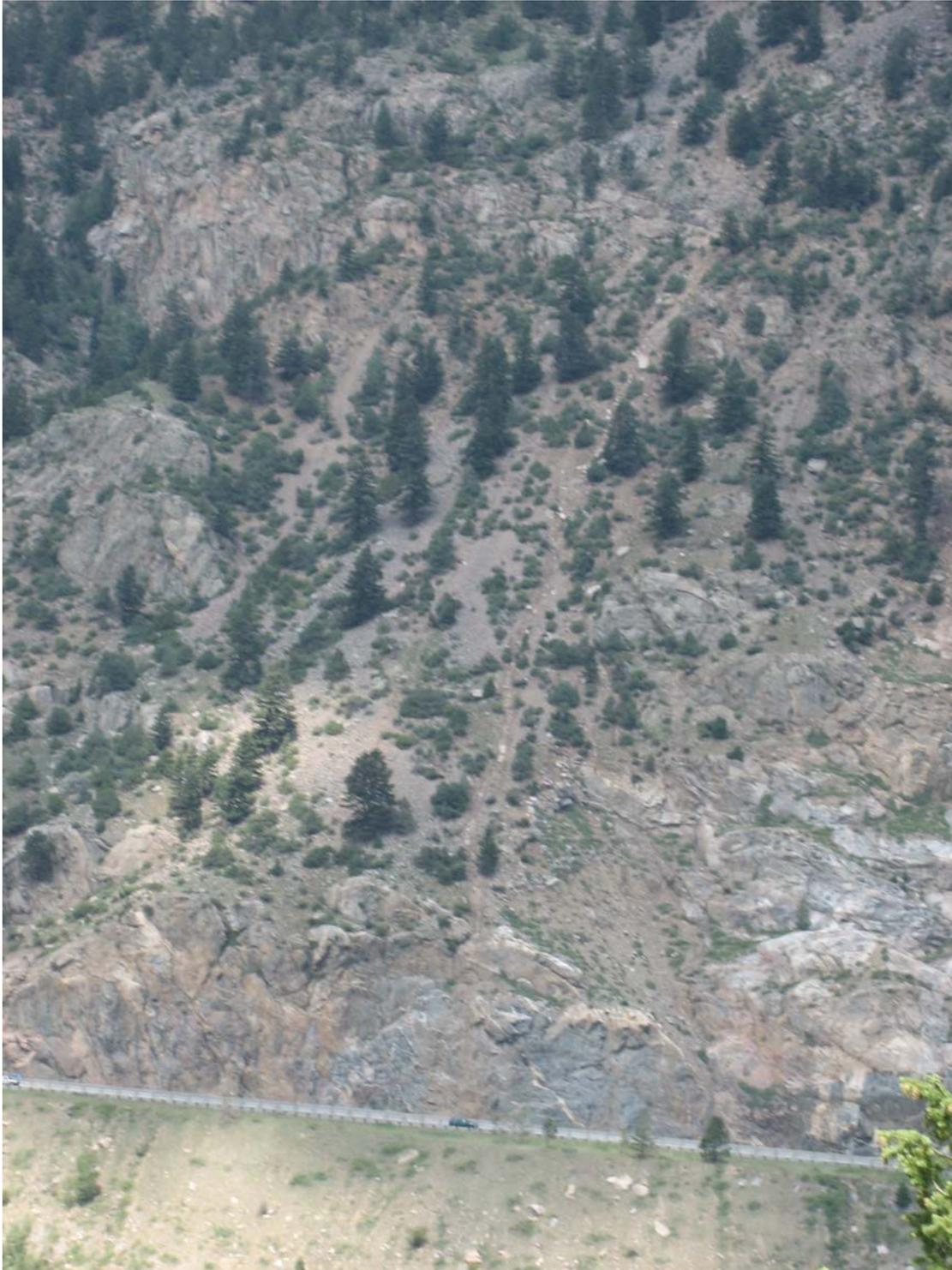
**Figure 18. Photo. Slope above the north side of Interstate 70 near Georgetown showing a small rockfall chute containing several large rock blocks.**
