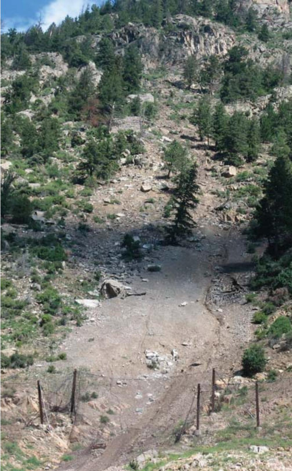
**Figure 17a. Photo. Rockfall chute, north side of Interstate 70 near Georgetown, Colorado.**
