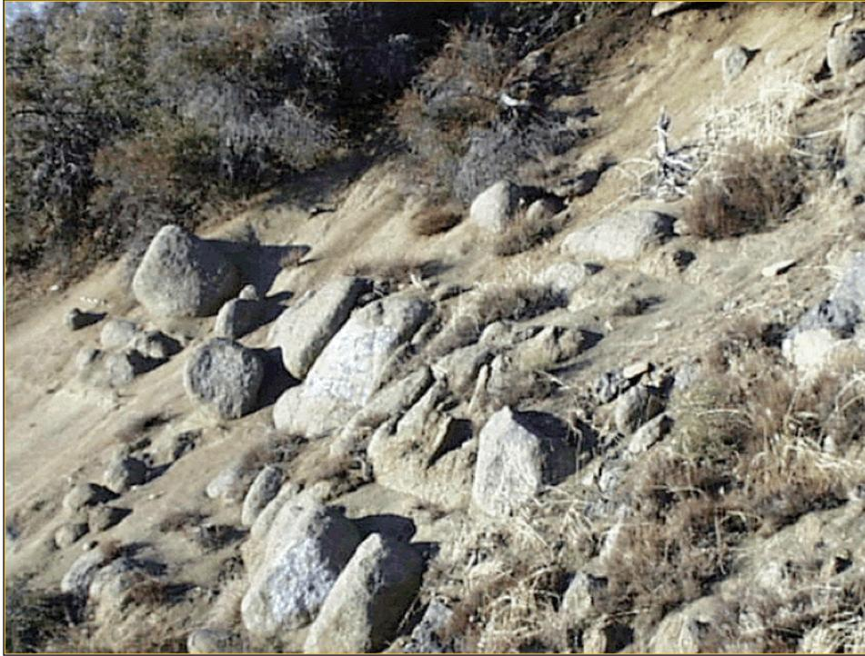
**Figure 16. Photo. Weathering of a slope near Pine Valley, California, exposing boulders that pose a rockfall hazard.**
