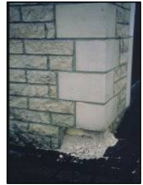
Figure 26: Stone destroyed due to frost
