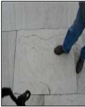
Figure 25: Cracks due to frost
