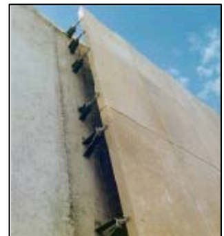
Figure 20: Traditional anchoring system with dowels
