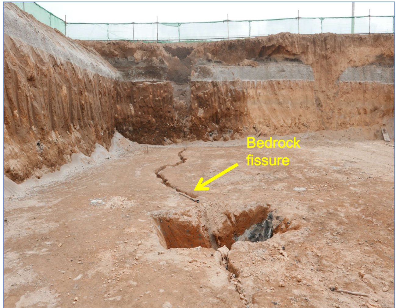
Earth fissure developed along bedrock fissure zone.
