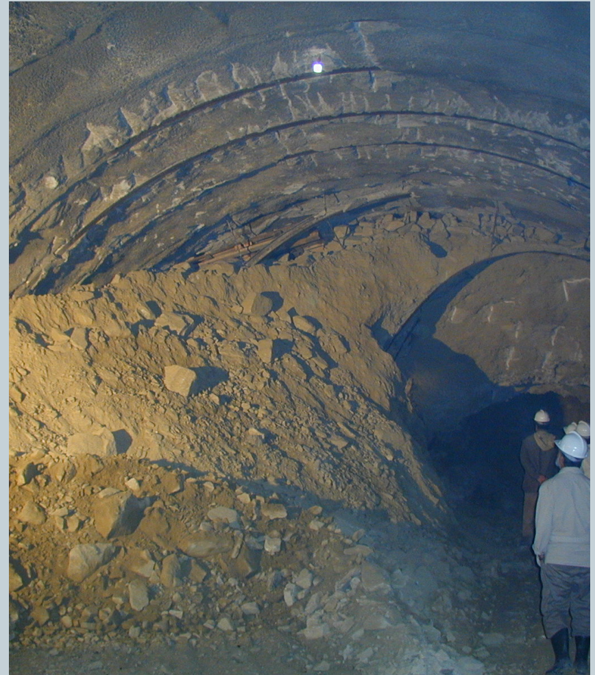
Chimney failure in highly weathered gneiss (Σ10 Tunnel, Egnatia Highway)
